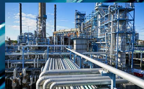
ORYX GAS TO LIQUID - QATAR UV systems for cooling water, reuse for irrigation
