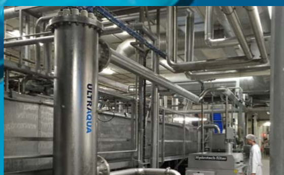
ARDO-FRIGODAN - DENMARK UV systems for recycled process water in the production of frozen vegetables
